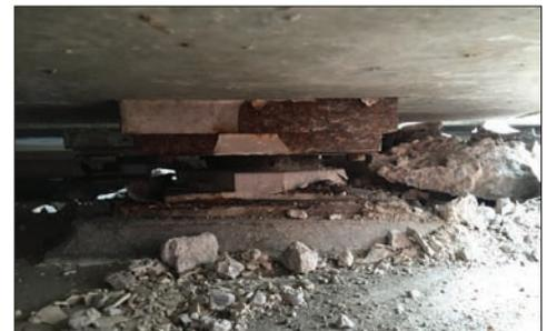
*Existing bearing showing excessive corrosion as a result of water leakage from the deck*
