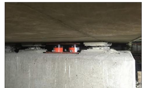
*Bearing shelf - localised jacking prior to bearing removal*
