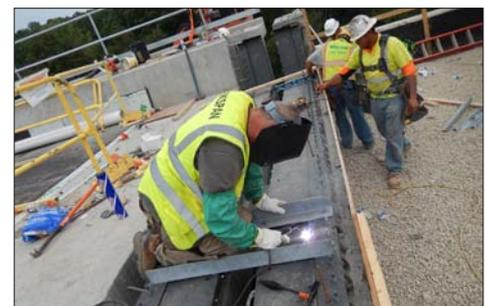
*Welding together of steel sub-structure plates*
