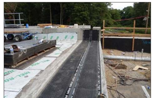
*West Abutment - New installed T-Mat 260 expansion joint*
